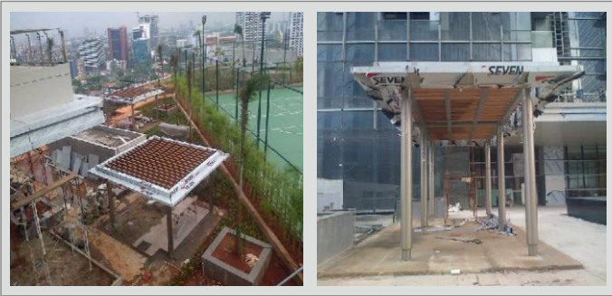
PROJECT CIPUTRA WORLD, CASABLANGKA - JAKARTA ( KANNOPY : ACP, KACA, & ENGINEERING WOOD )
