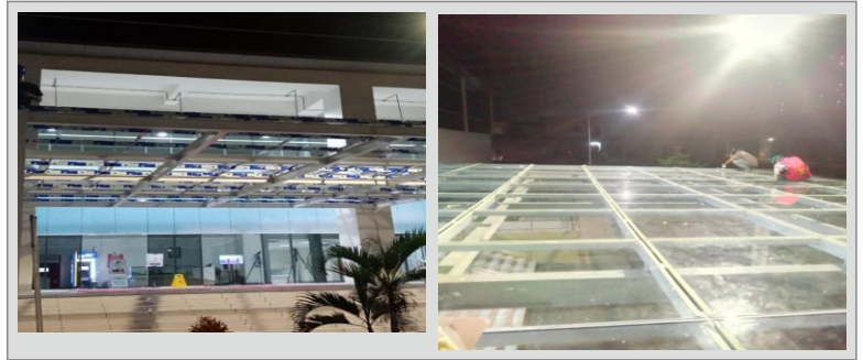
PROJECT LRT, KELAPA GADING - JAKARTA ( KANNOPY KACA )
