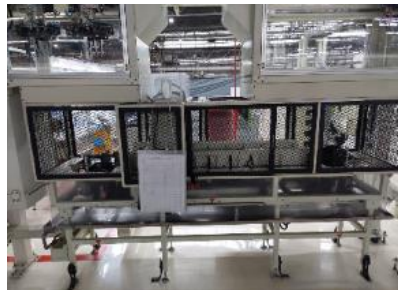
Buffer Conveyor (PT. Astra Daihatsu Motor)
